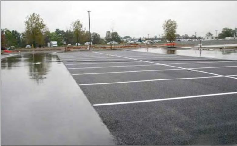
Resurfacing on Second Street will utilize permeable asphalt, similar to what is pictured above. Permeable asphalt captures stormwater rather than allowing it to run off into vulnerable water sources. This method of street design mitigates erosion while improving water quality. The use of permeable asphalt should be considered in future street improvements when appropriate.
