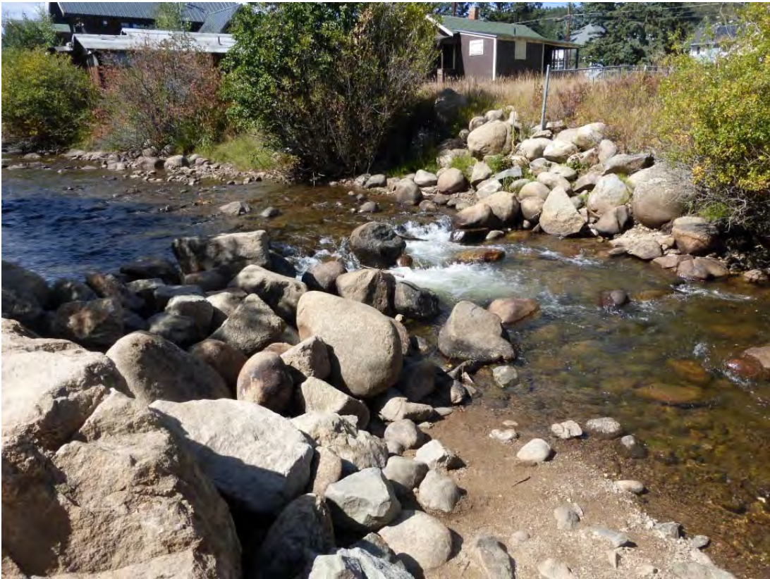
Photo 12. Rock check dam below homes pictured in Photo 11.
