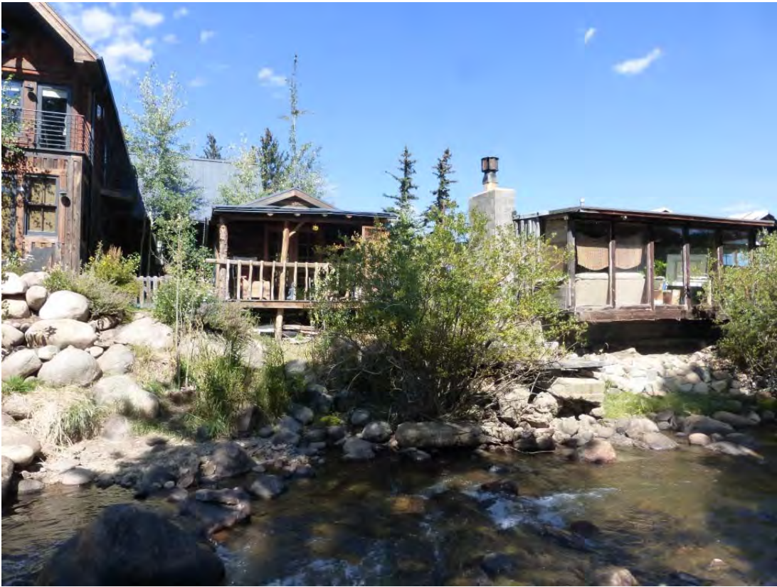
Photo 11. Bank instability along homes on north side of Middle Boulder Creek.
