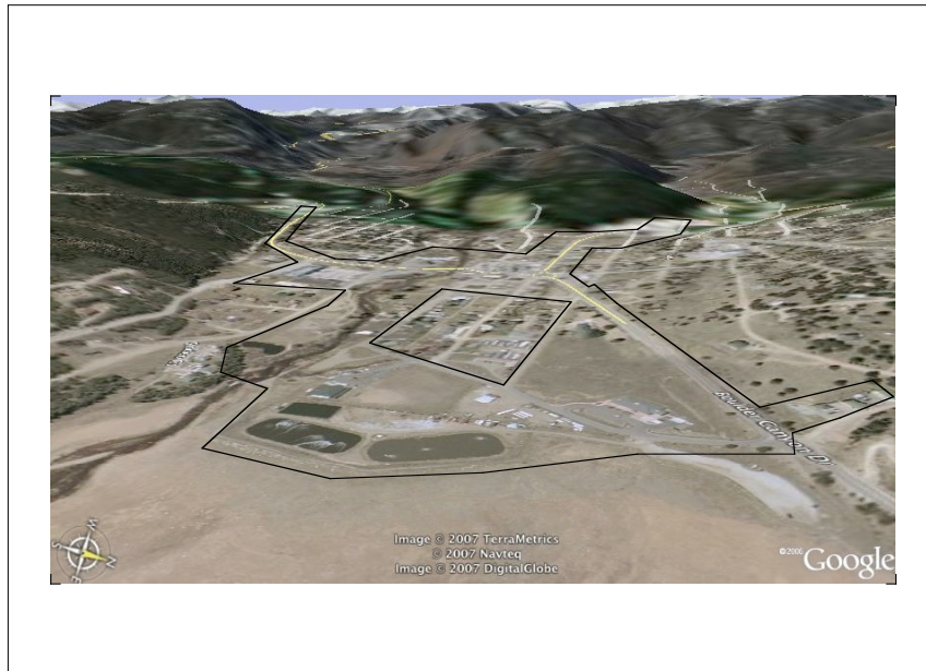
View of Nederland from the East With the Downtown Development Area (approx)
