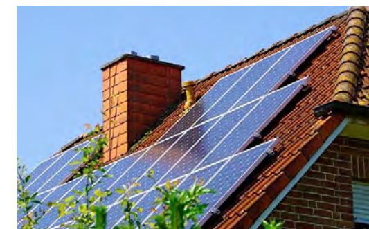
ROOFTOP SOLAR PANELS
